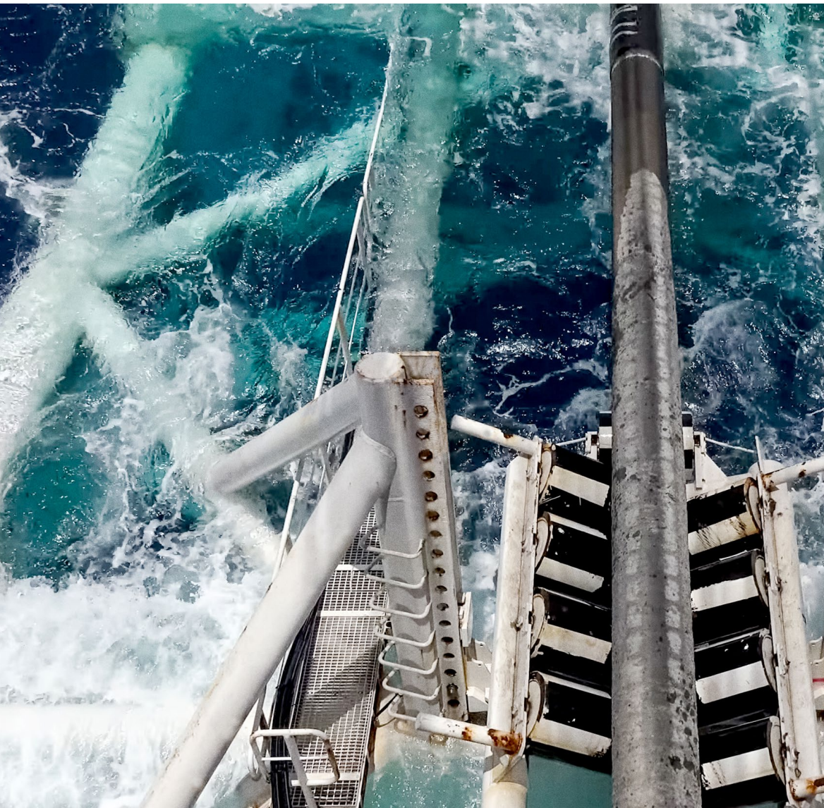
Figure 1. Laying an offshore gas pipeline on the seabed.
